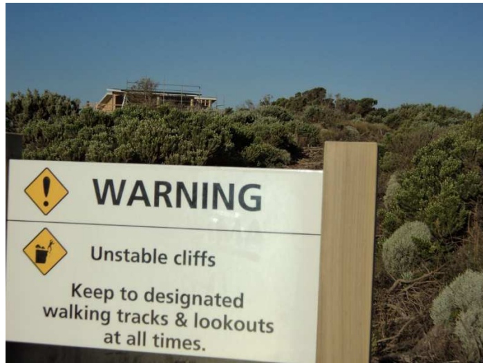
Building near unstable cliffs and large caverns and tunnels
