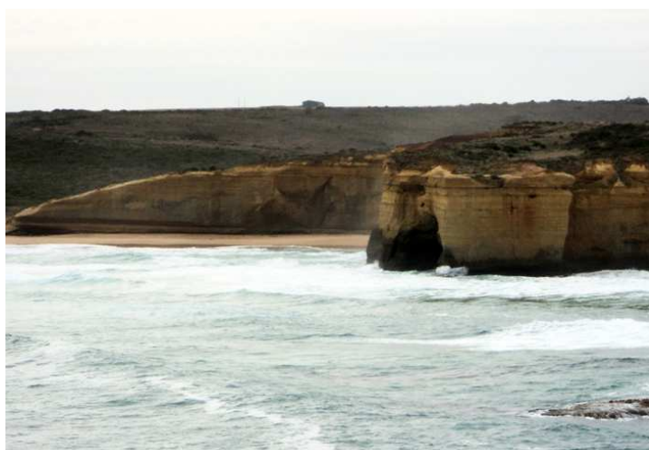
Sheds disrupt scenic lookout and important hinterland viewlines and Great Ocean Road viewlines
